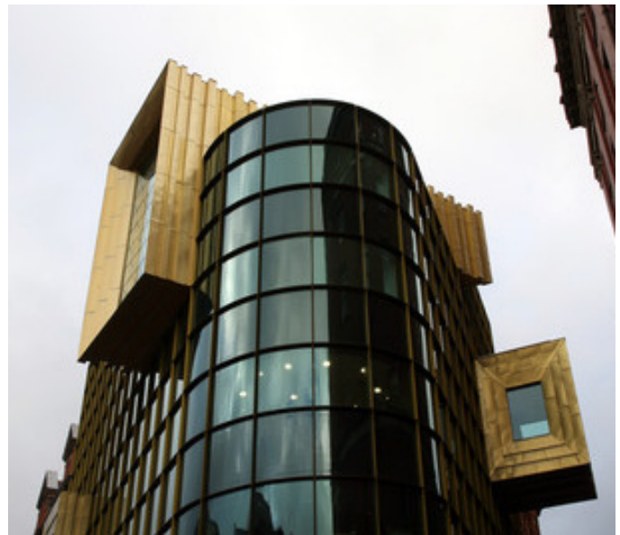
Liverpool City Council and Construction Partners sought to deliver the comprehensive redevelopment of approximately 42 acres at the heart of Liverpool's existing retail core and World Heritage Waterfront.
